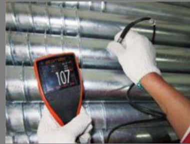
Steel Structure Film Thickness Test
